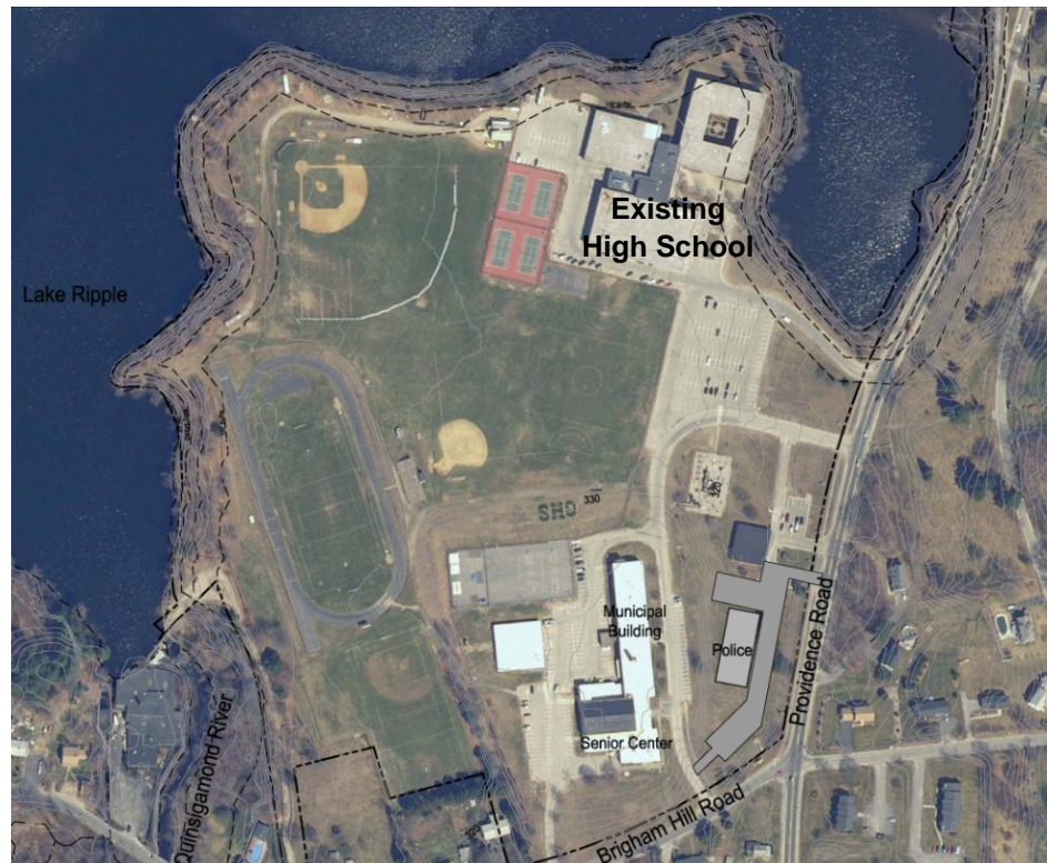
Figure 3.A: Existing High School Site
