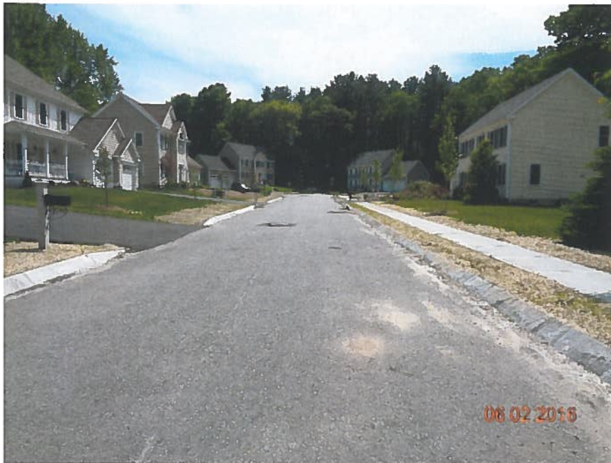
Desrosiers Landing, looking south into the project.
