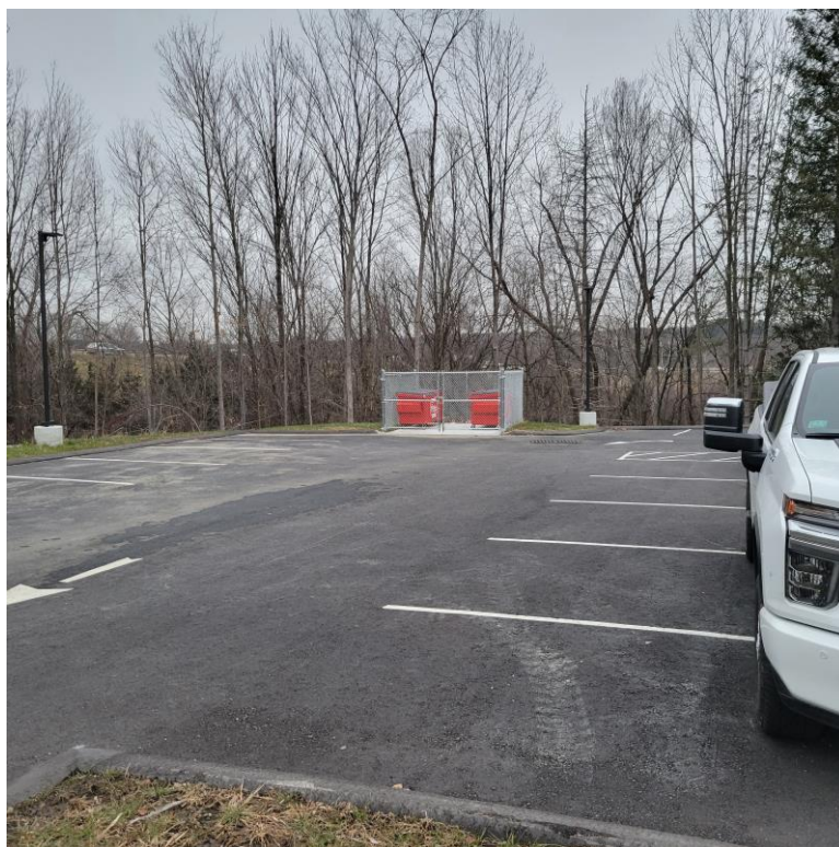
Photo 2: Dumpster enclosure with fencing installed.
