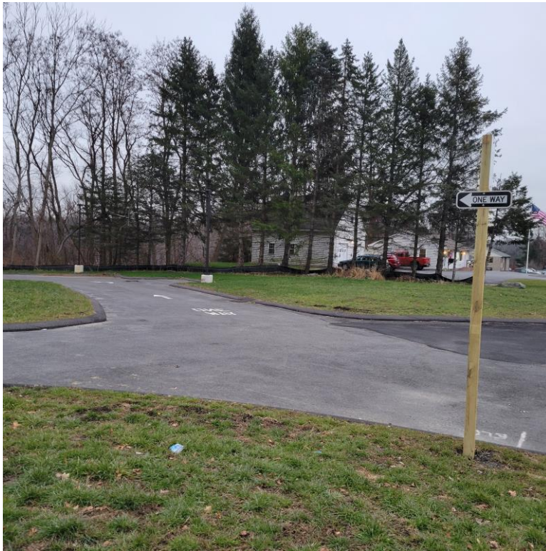
Photo 4: General condition of driveway entrance with pavement markings and temporary signage.
