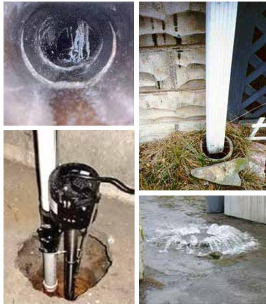
sewer infiltration (top left), roof gutter connection (top right), sump pump (bottom left), sewer overflow (bottom right)
